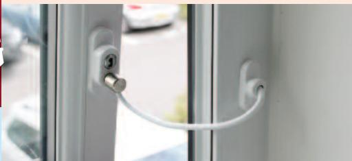
The window restrictors installed may be inadequate to prevent a determined force to open a window beyond the 100mm restriction.
